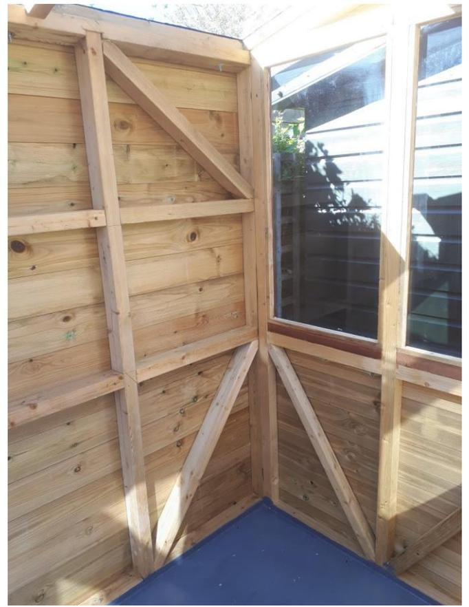
Strongly constructed of 3" x 2" structural treated timbers with wind bracing
