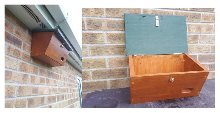
All paint finished both internally and externally with two coats of Sadolin exterior antique pine wood stain and roof with forest green Ducksback preparation to afford maximum weathering.
