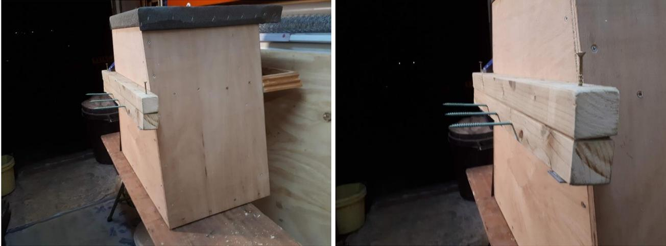
Constructed of 2 no. 47 x 47mm treated timber sections; one bolted to the Owl box, the second (tree plate) to be mounted horizontally and centrally on the tree trunk at a height of at least 3 meters above ground using 3 no. 7 x 150mm heavy duty timber drive screws (supplied). It has 2 no 50 x 100mm galvanised mild steel angle brackets attached.
